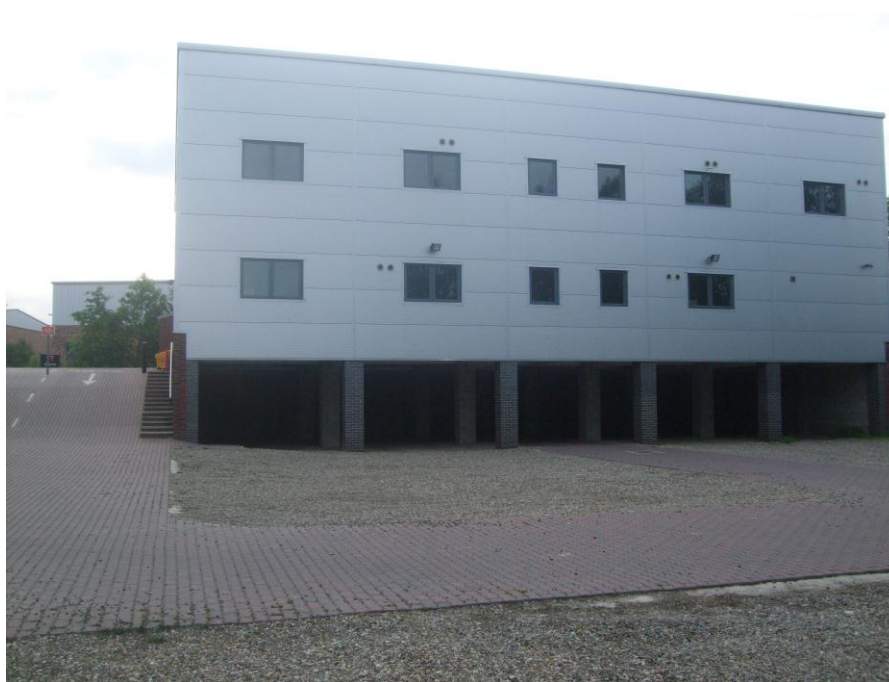
Rear elevation of existing building
