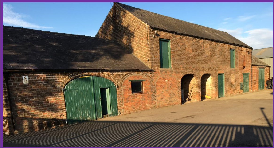
Photograph taken prior to conversion works
