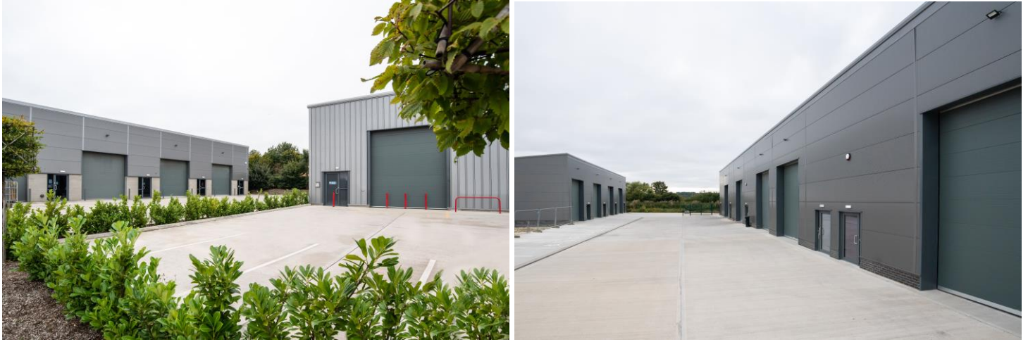
New Commercial Units already built and occupied.
