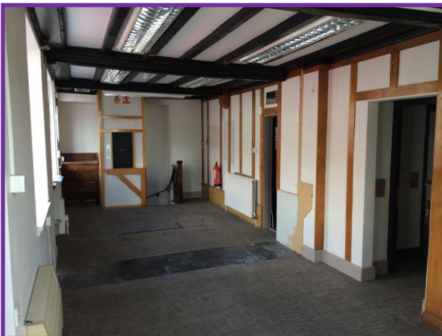
Internal prior to most recent tenant
