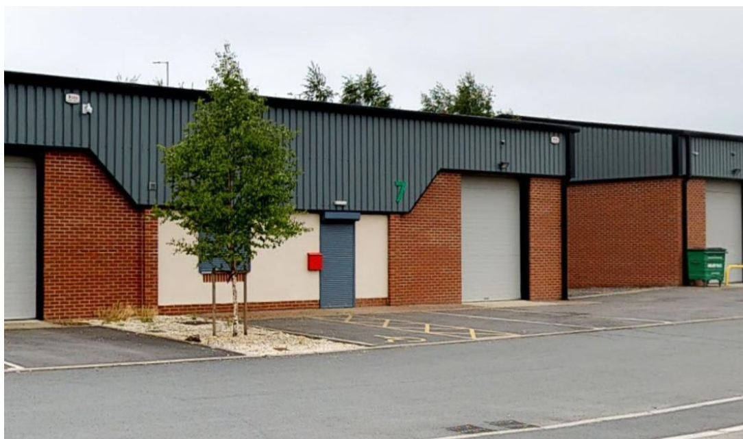
Original photo after construction
